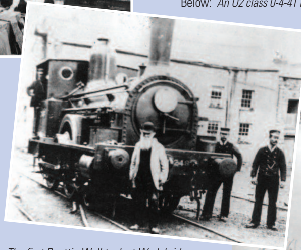
The first Beattie Well tank at Wadebridge was 248 which arrived in June 1893 and departed to Nine Elms in May 1895. This loco was withdrawn in December 1898. Wharfinger Sam Worth poses with staff in front of this loco at Bodmin Wharf.
